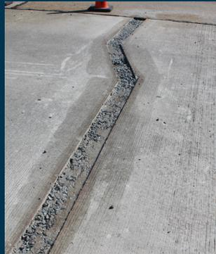
Pour molten Fibrecrete G into the remaining repair depth, screed to a level grade and apply Topping Stone for skid resistance.
