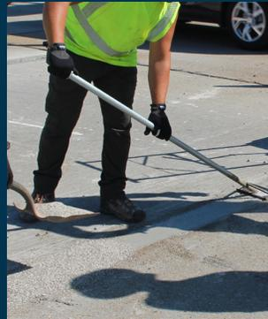
Allow Fibrecrete G repair to cool and reopen to traffic, usually within an hour depending on the size of the repair.
